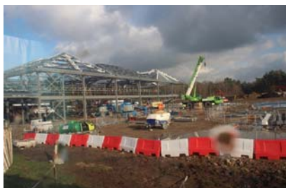
The new entrance building under construction.
